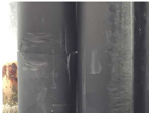
Figure 6: Close up of damage
