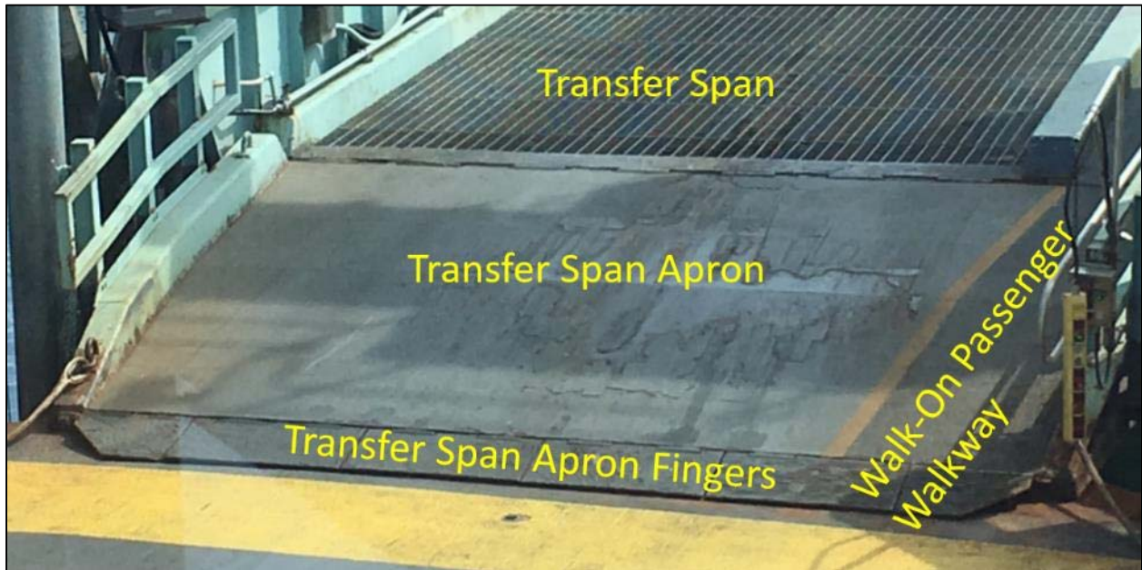
Figure 9 Transfer span components
