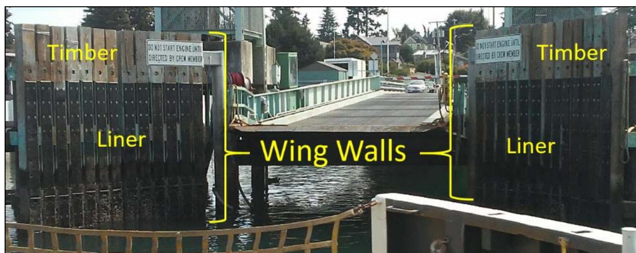
Figure 8 Wing walls at Anacortes terminal
