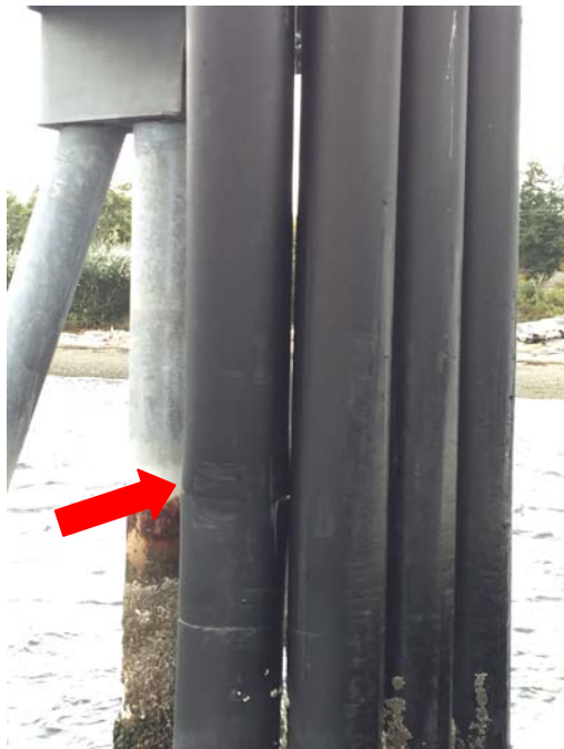
Figure 5: Damage to Guemes Dolphin 'C'
