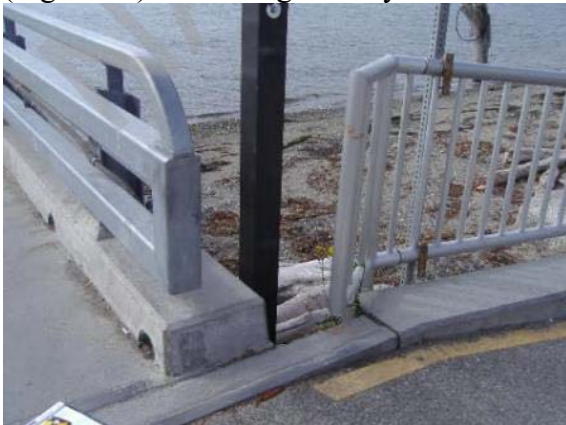
Figure 15 Non-compliant gap at Guemes Island terminal (Source: Reference 5)
